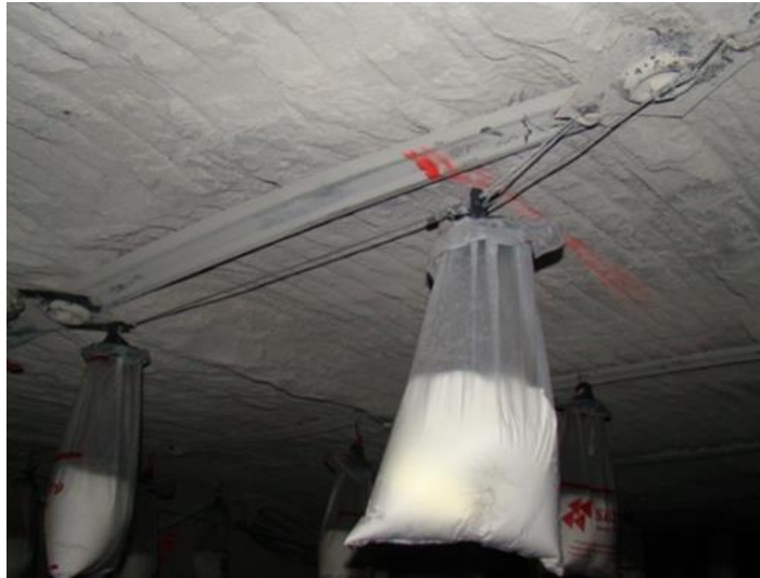
Figure 4.4: Cable and Hook Support Method
